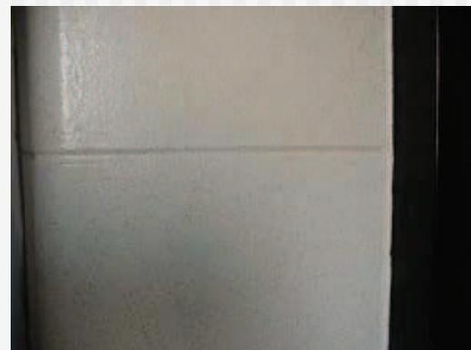
◀ Block Wall - Filled and Spatter Coated
